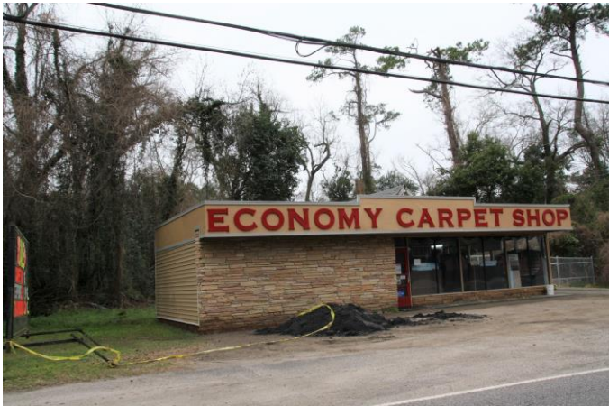
SITE – The Jessamine Apartments 421 Cashua Drive, Florence, SC Facing west from Cashua Road Existing commercial building on site to be razed
